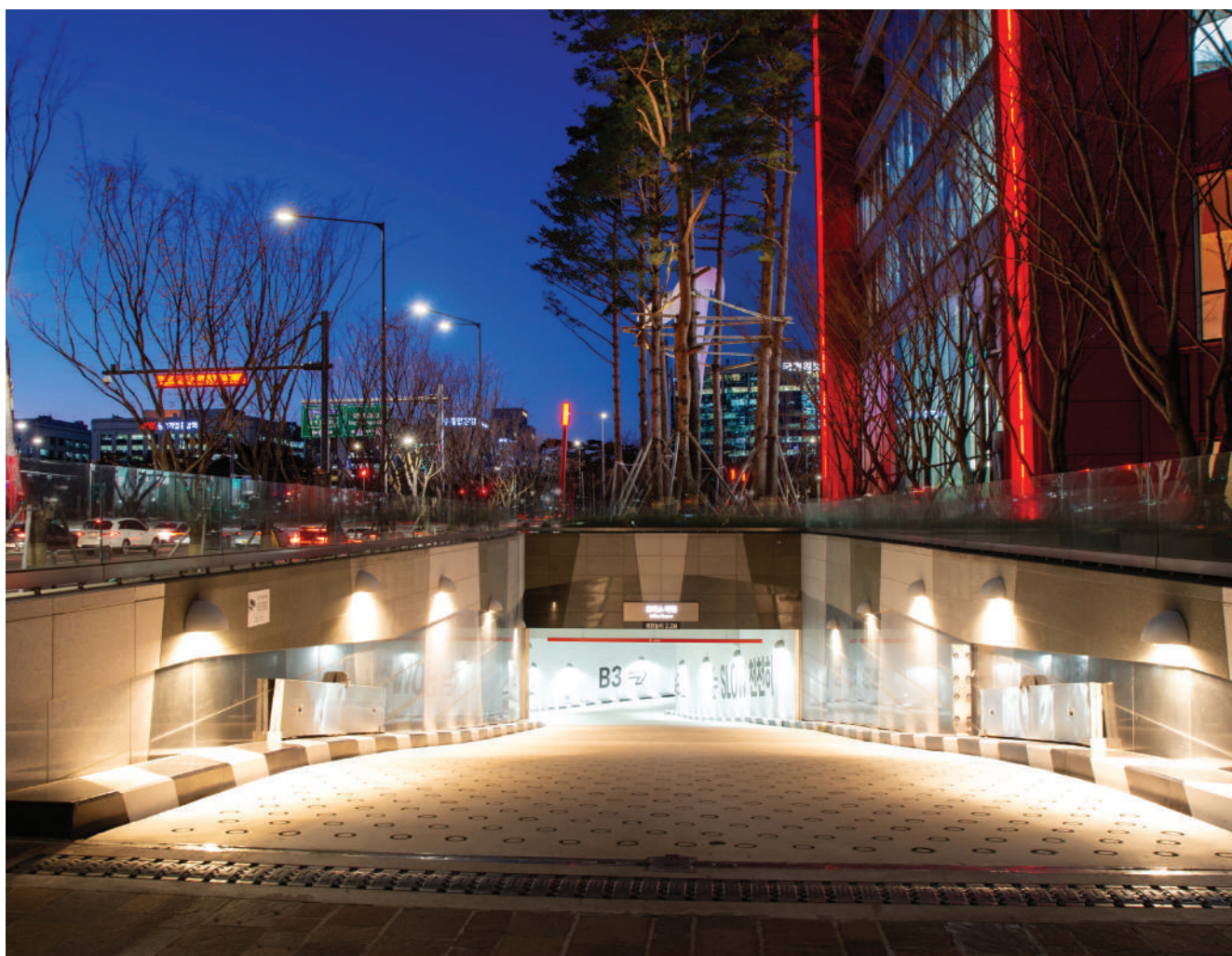
Parc.1 tower, Seoul
