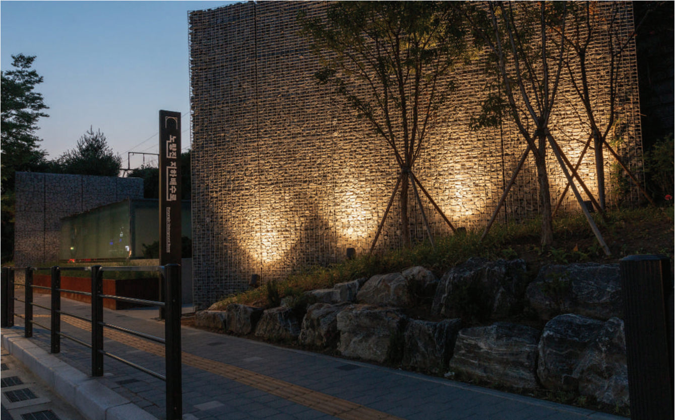
Noryangjin Underground Sewer
