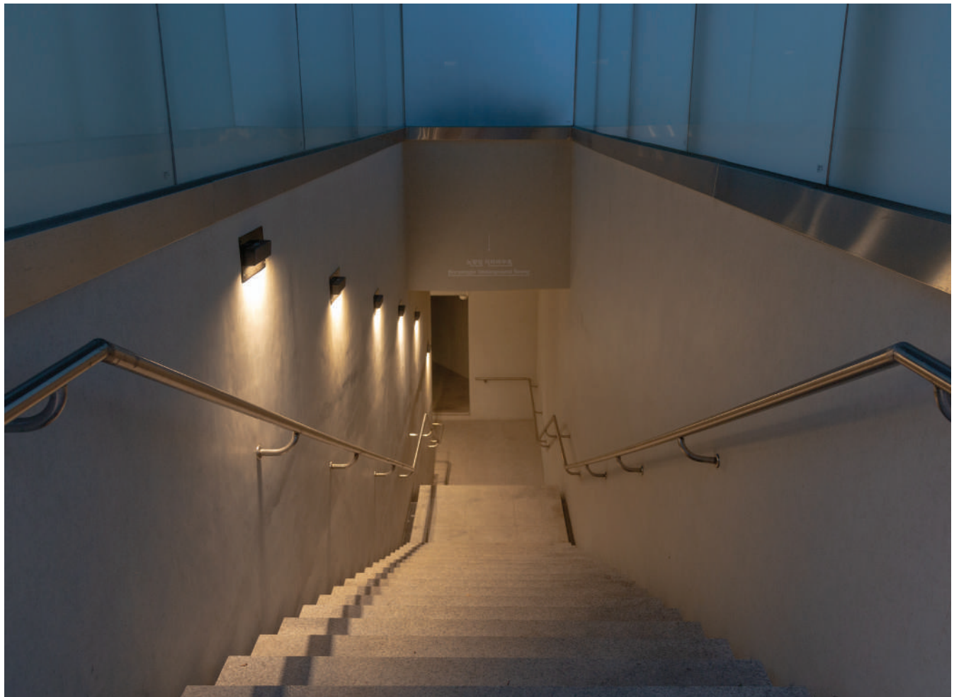
Noryangjin Underground Sewer
